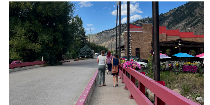
Bellm Bridge links Minturn's 100 Block and the municipal parking lot.
