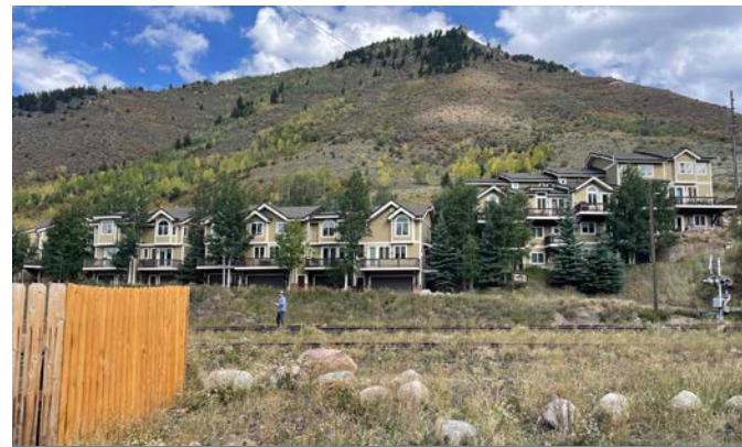
Newer construction in Minturn.
