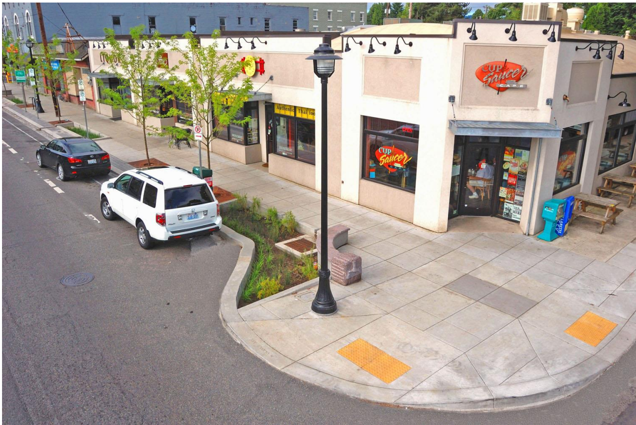
Figure 6: Example of a Curb Extension – Portland, OR (Source: GreenWorks)
