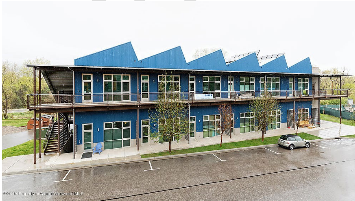
Live-work development near Basalt, Colorado allows light industrial, professional, and residential uses.
