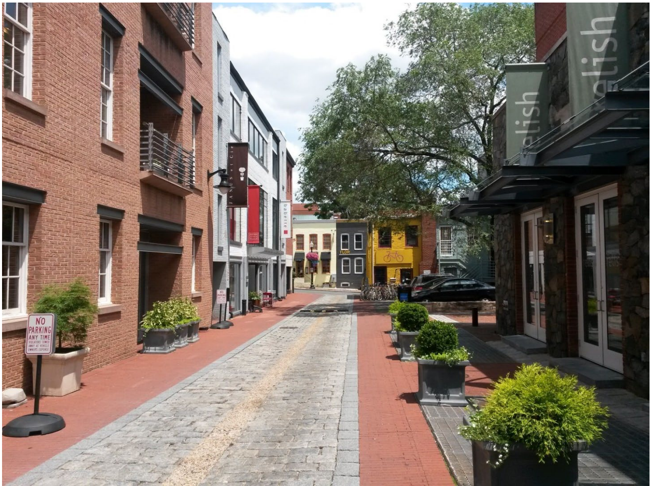
Figure 7: Example of a Shared Street – Cady's Alley, Georgetown, Washington D.C. (Source: Martinez and Johnson Architecture)
