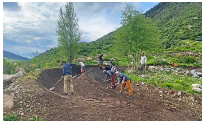
VVMTA seasonal crews work on bike trails (VVMTA)
