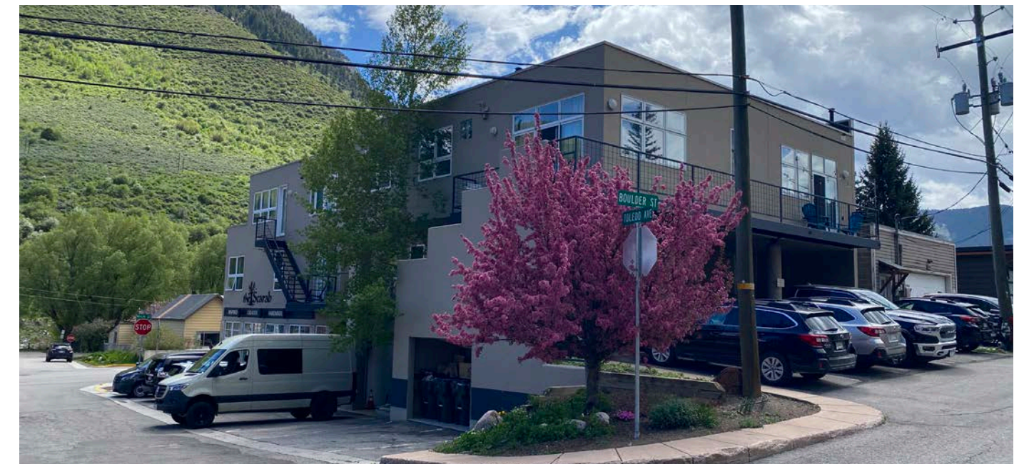
The Scarab is an example of an existing mixed-use building in Minturn.
