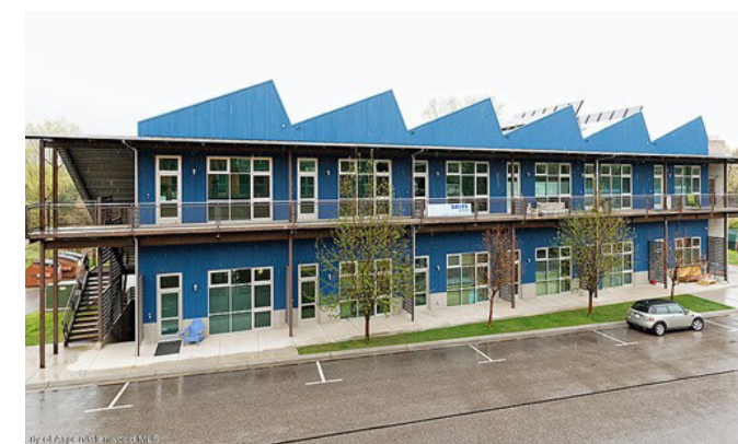
Live-work development near Basalt, CO allows light industrial, professional, and residential uses.
