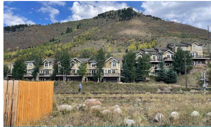
Newer construction in Minturn.
