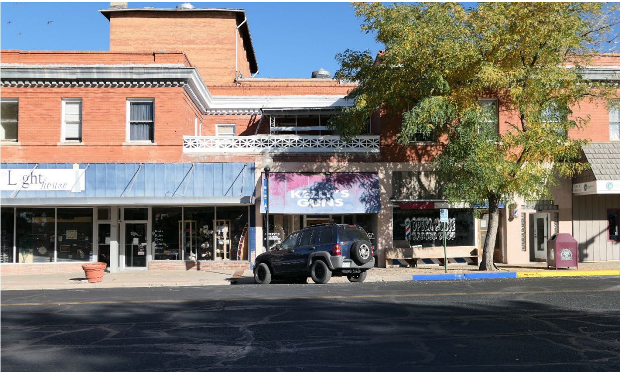
5OT-1721_215 Colorado Ave_03 West side, center
