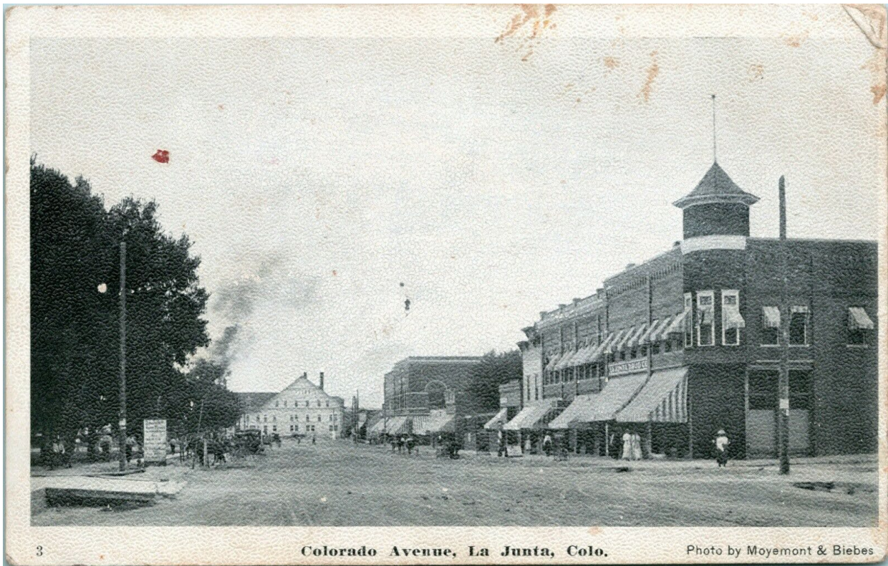
Figure 2: East side of Colorado Avenue ca. 1906 after completion of the second floor of the Pierce Block (far right). La Junta Theatre and E.W. Pierce's two-story wood-frame commercial building adjacent to the north. (Postcard/ebay.com)
