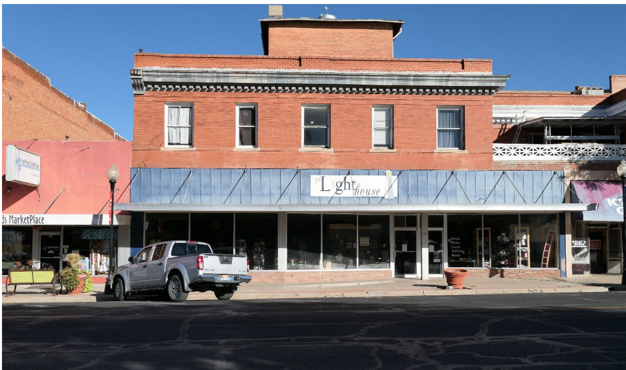
50T-1721_215 Colorado Ave_02 West side, north half camera facing east
