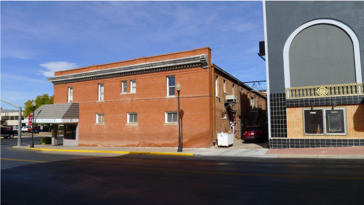
5OT-1721_215 Colorado Ave_06 South and east sides
