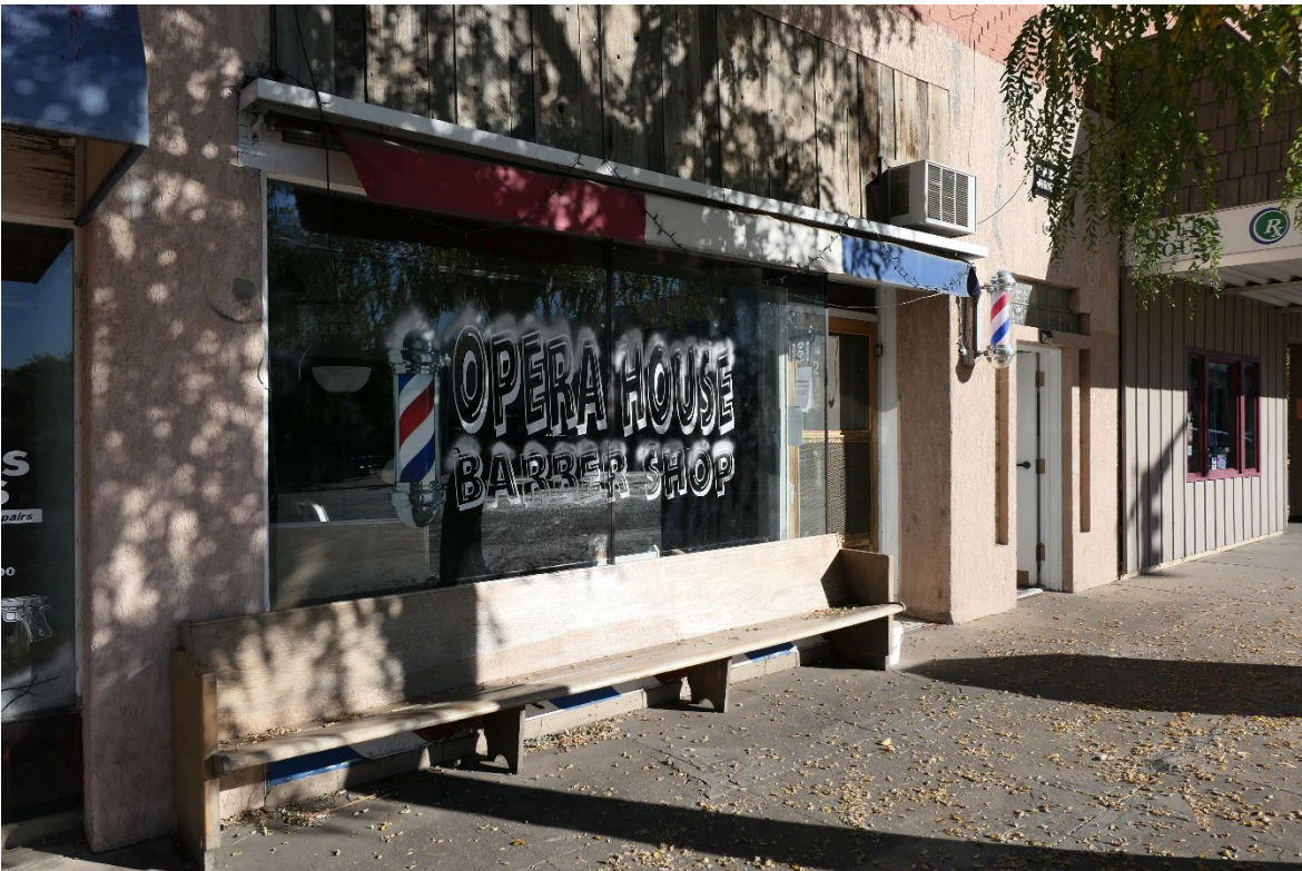
5OT-1721_215 Colorado Ave_09 Detail of south center storefront and upstairs entrance camera facing southeast
