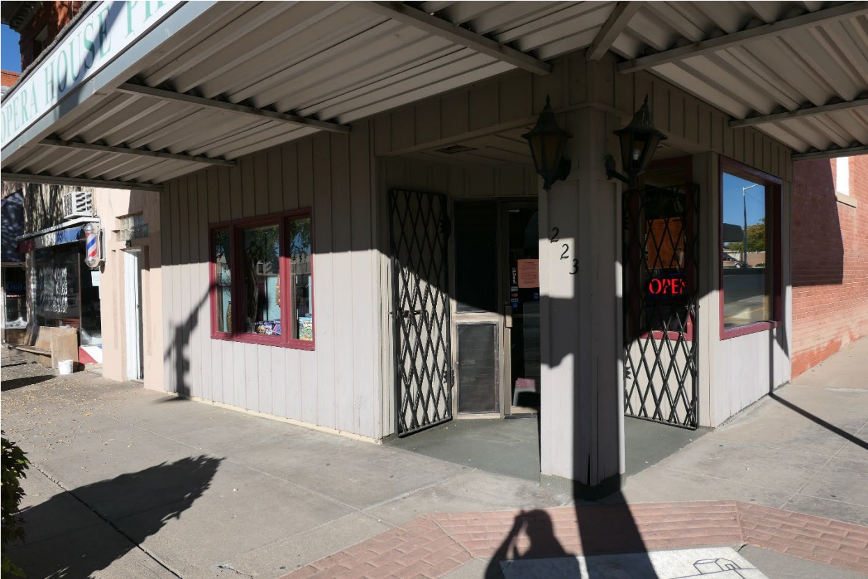
5OT-1721_215 Colorado Ave_08 Detail of southwest corner storefront
