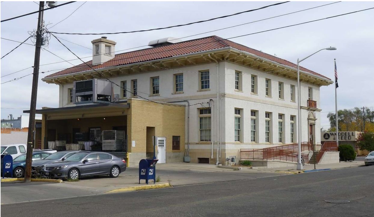
5OT94_324 Colorado Ave_02 West and south sides camera facing northeast
