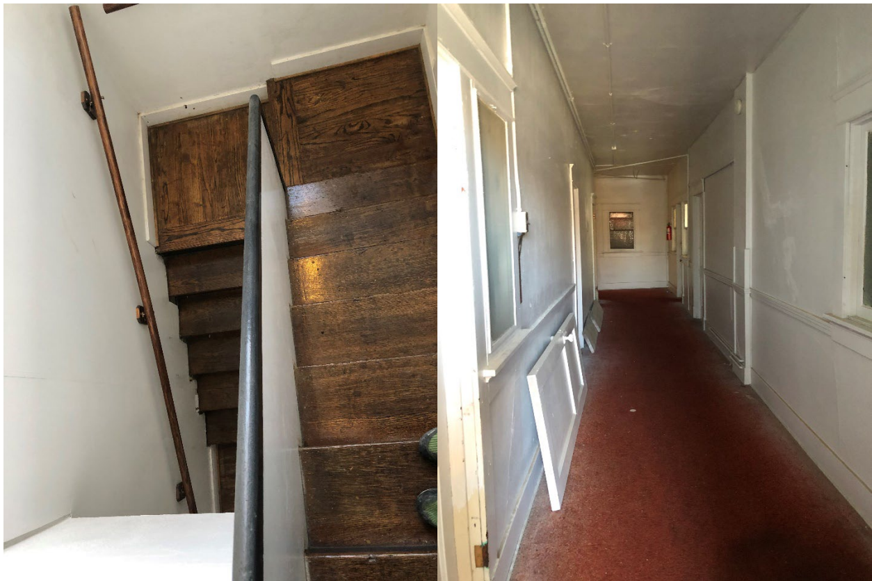
Figure 24: Stairway to second floor apartments and second floor hallway in 2019. (Preliminary Property Evaluation Form, 5OT.1721/History Colorado)
