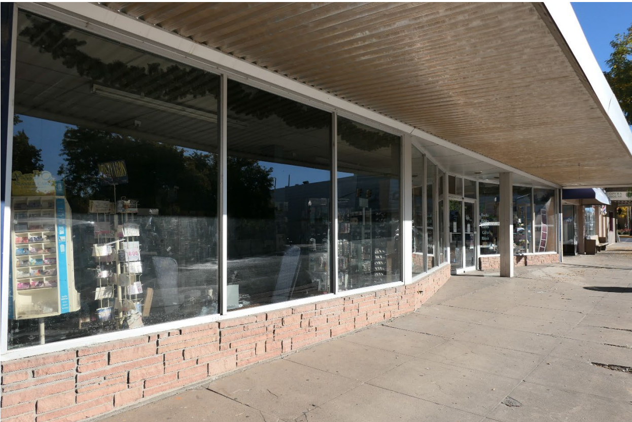
5OT-1721_215 Colorado Ave_11 Detail of north storefront
