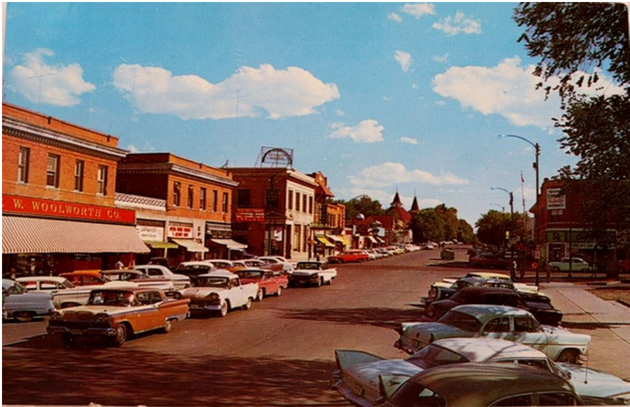
Figure 15: Opera House Block ca. 1950s-early 1960s. (Woodruff Memorial Library)
