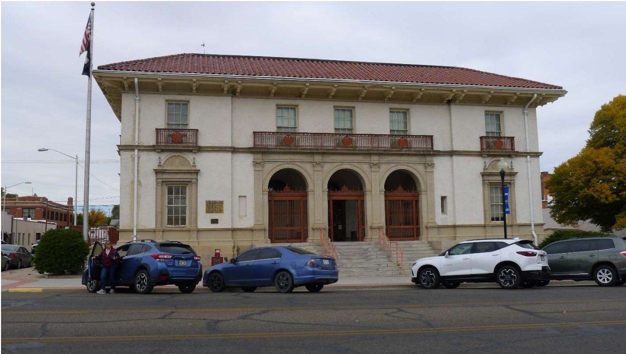
5OT94_324 Colorado Ave_01 East side camera facing west
