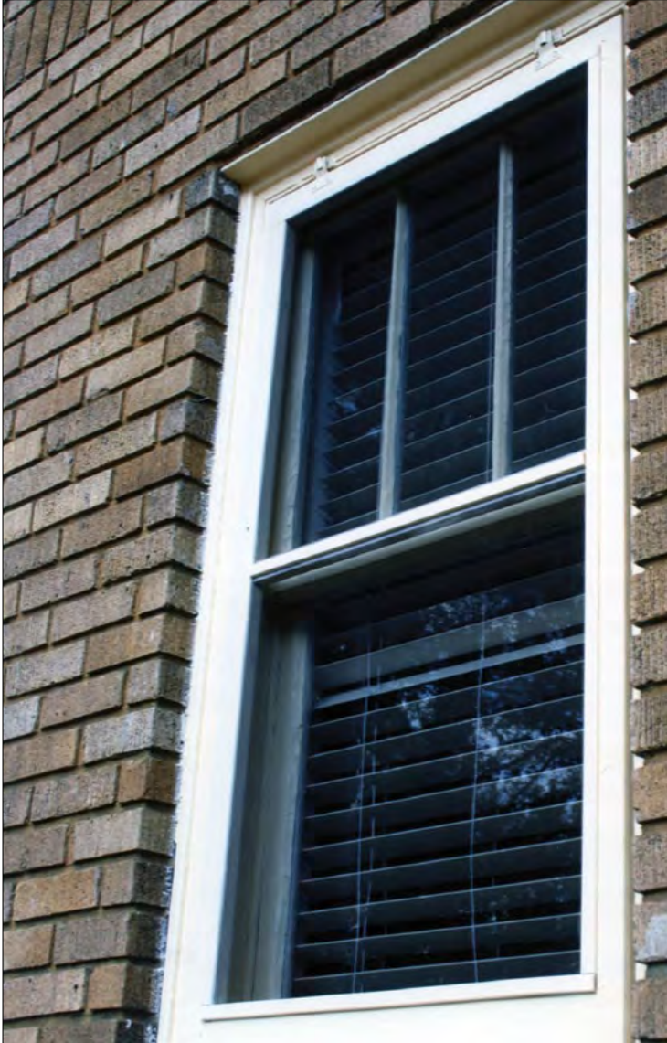
[10] Historic exterior storm windows preserve and help to insulate wood windows.
