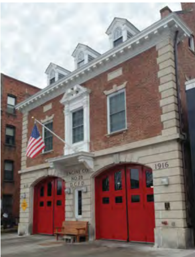
[56 a-b] In order to continue in its historic use, the door openings of this 1916 Colonial Revival-style fire station had to be widened to accommodate the larger size of modern fire trucks. Although this resulted in some change to the arched door surrounds, it is minimal and does not negatively impact the historic character of the building. (a) Above, before; Photo: Fire and Emergency Medical Services Department (FEMS), Washington, D.C.; below, after.
