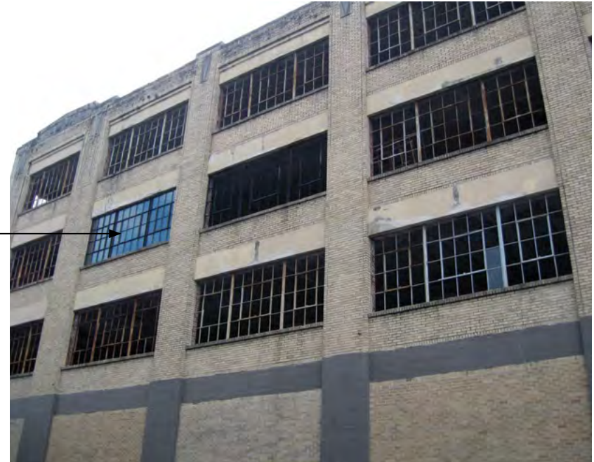
[19] Installing a mockup of a proposed replacement window can be helpful to evaluate how well the new windows will match the historic windows that are missing or too deteriorated to repair.
