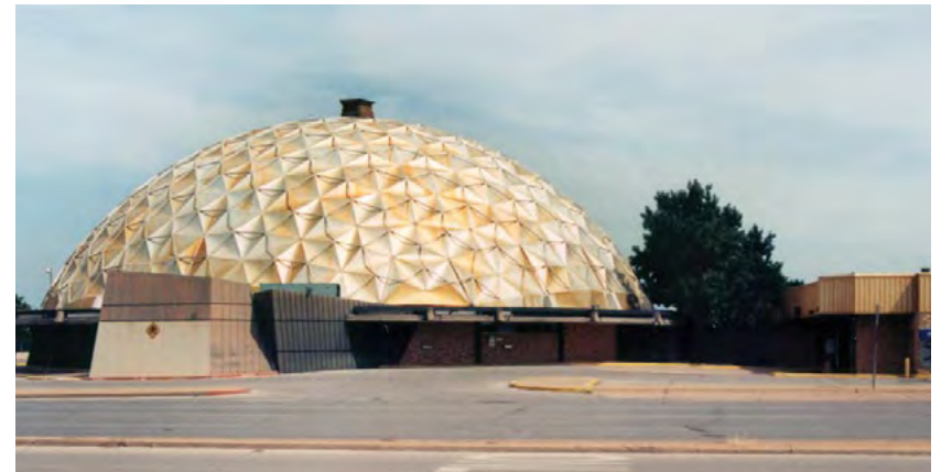
[13] The gold-colored, anodized aluminum geodesic dome of the former Citizen's State Bank in Oklahoma City, OK, built in 1958 and designed by Robert Roloff, makes this a distinctive mid-20th century building.
