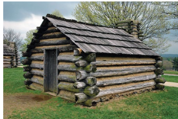
[7] The Muhlenberg Brigade Huts are reconstructions of nine log huts erected in 1777 at Valley Forge during the Revolutionary War. They have been reconstructed on the historic road with logs cut with modern power tools and finished with cement, unlike the original logs which were hand hewn and finished with traditional chinking. Photo: Rdsmith4 at Wikimedia Commons.
