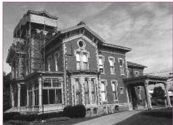
Kalamazoo, Michigan American Red Cross Restoration Project
