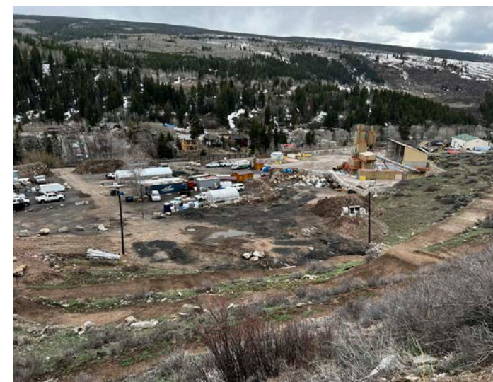
Public Works Facility view from the Mini Mile
