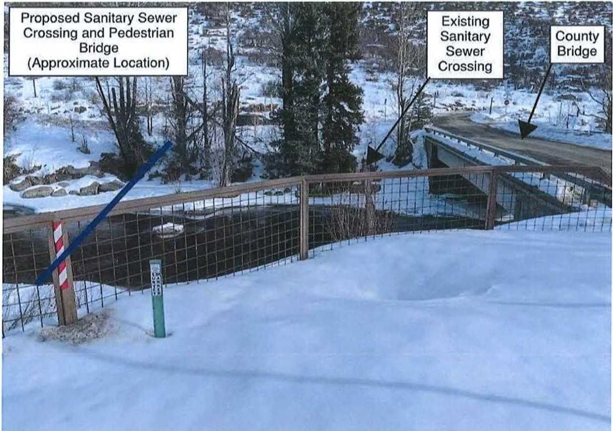
This photo is taken from the Eagle Valley Trail looking across the Eagle River at the project site.
