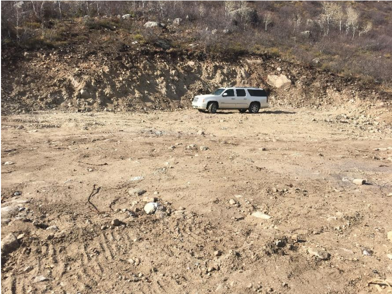
Preliminary Water Tank Platform
