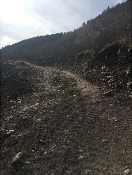
Water tank road
