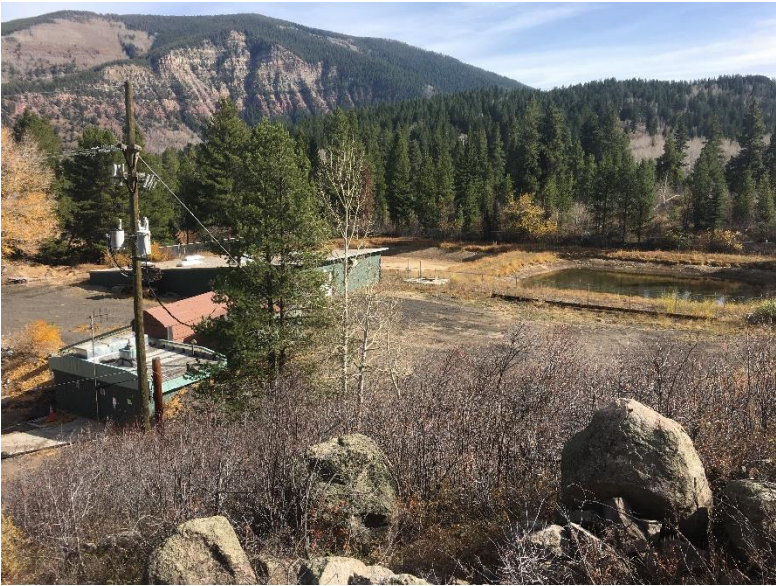
Existing Water Treatment Plant
