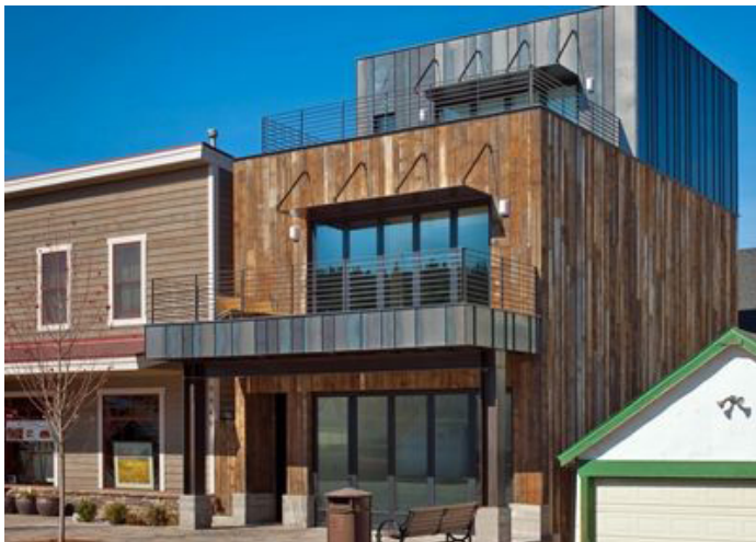
A modest 3-story mixed use building.
