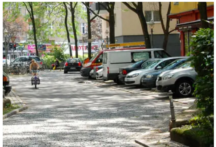
90-degree parking in the rear setback along Williams (south of Nelson Avenue) is required.
