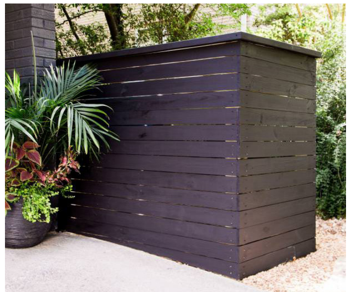
All refuse storage shall be 6-foot tall if detached from the primary structure and designed with high-quality materials.
