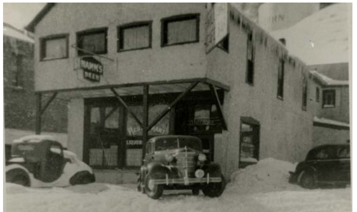
The Williams Cafe and Bar (now Magustos) is a wood and stucco structure that includes an arcade and storefront.
