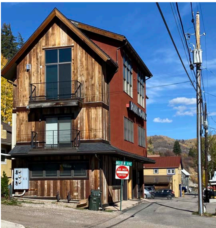
Hotel Minturn is a local example of a taller-than-average building that fits in nicely due to the massing, roof design, and materials.
