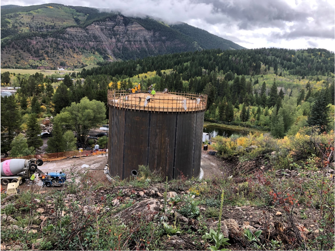
Figure 5 – Forming of dome roof
