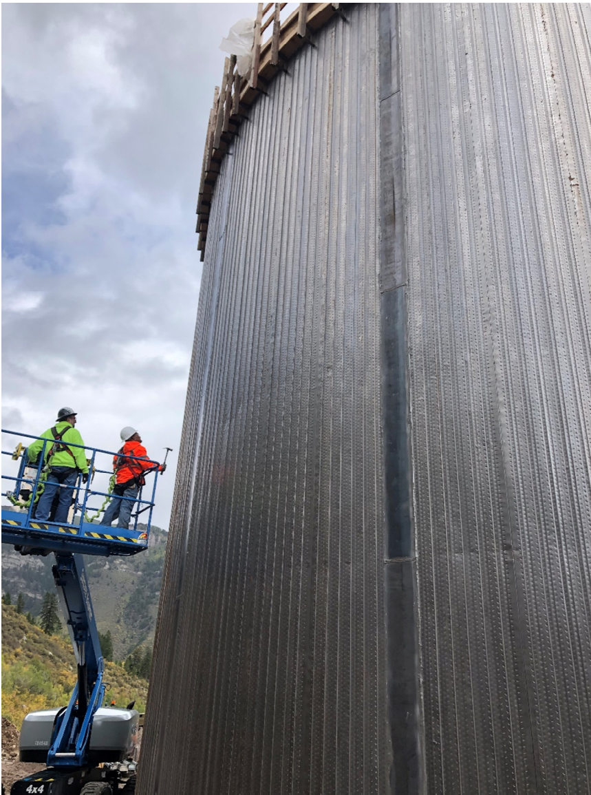
Figure 1 – Wall gap metal supports
