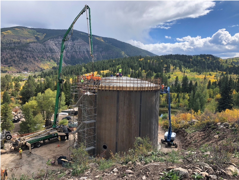
Figure 1 – Pouring roof
