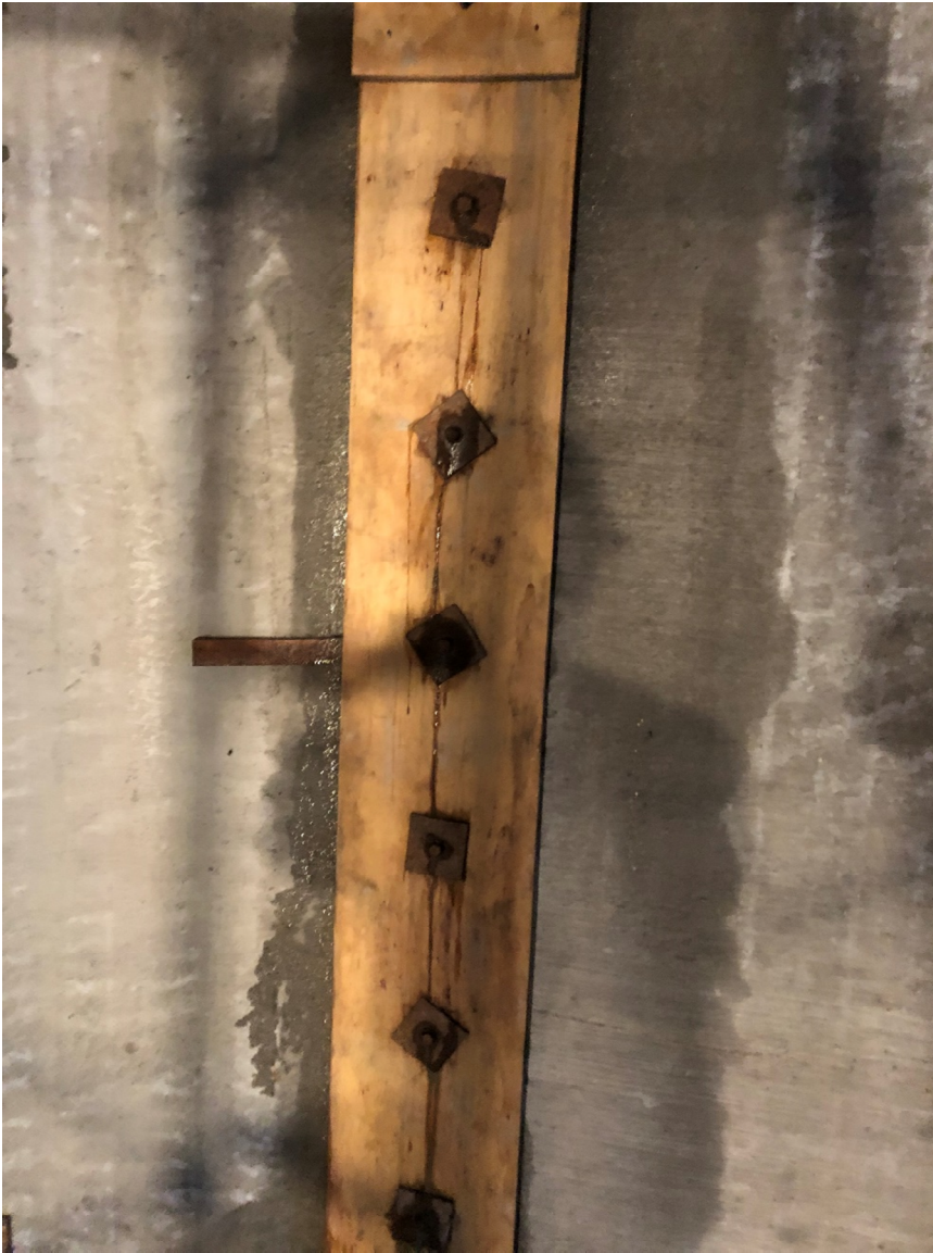
Figure 4 – Wood backer at wall slots
