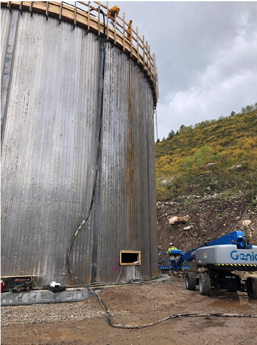
Figure 2 – Pumping concrete for wall slots
