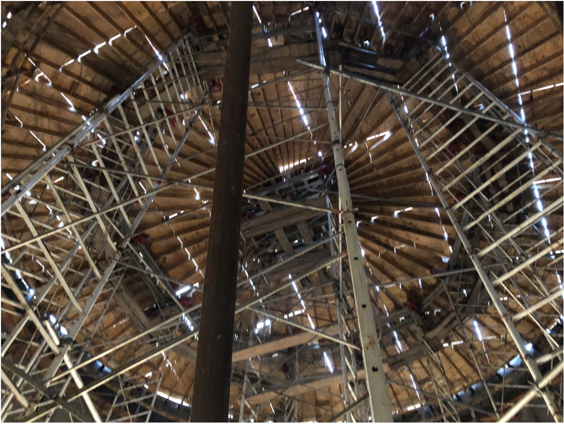
Figure 3 – Scaffolding and formwork for domed roof
