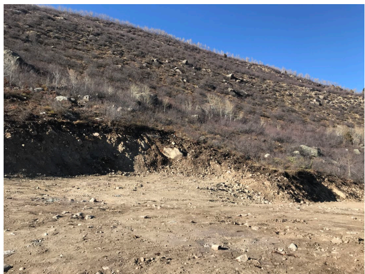
Partial view of water storage tank pad, still under construction.
