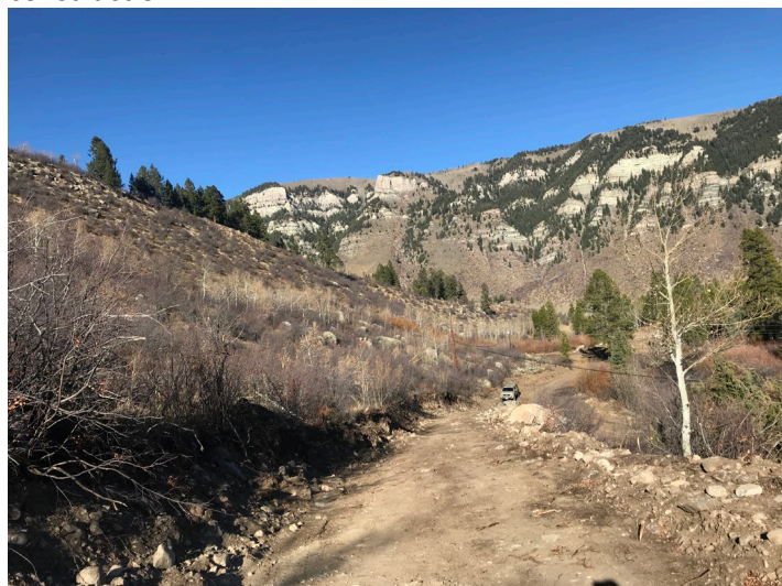
View looking down access road from pad site, still under construction.
