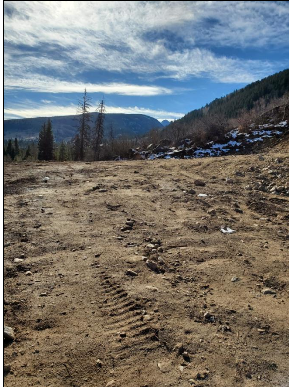
Overview of water tank location from access road, facing south (Roll 20-104, unaltered image 01, 11/22/2020)
