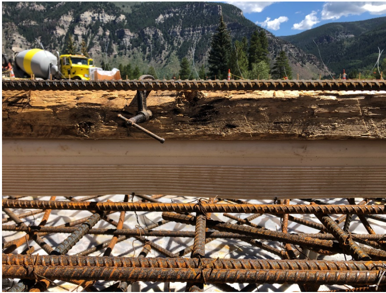
Figure 4 – Tank waterstop
