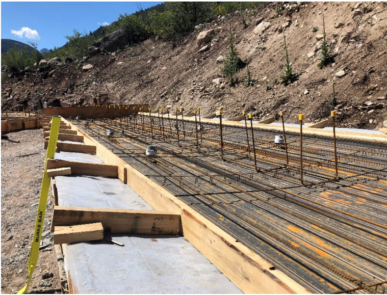
Figure 2 – Wall panel with reinforcement for overflow piping
