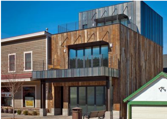
A modest 3-story mixed use building.
