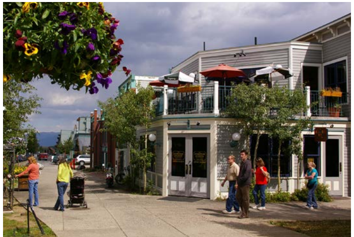
Designing at a human scale means designing a building that is comfortable for someone to stand by and be in.
