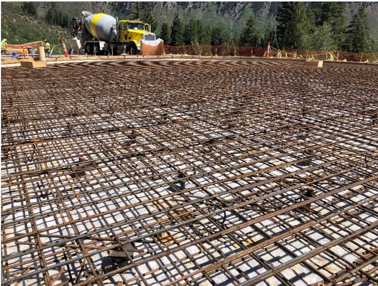
Figure 3 – Tank floor rebar layout
