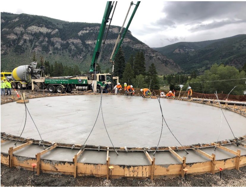
Figure 6 - Finished Tank Floor
