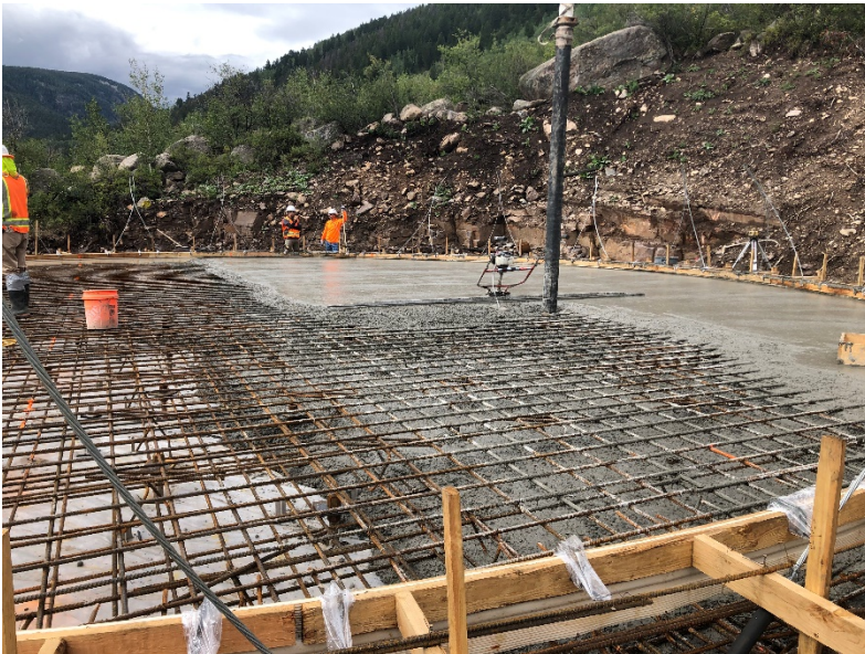
Figure 5 – Pouring concrete
