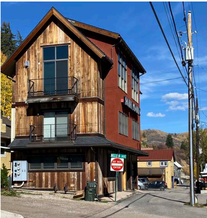
Hotel Minturn is a local example of a taller-than-average building that fits in nicely due to the massing, roof design, and materials.
