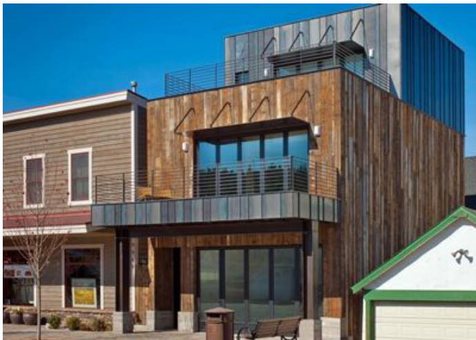
A modest 3-story mixed use building.
