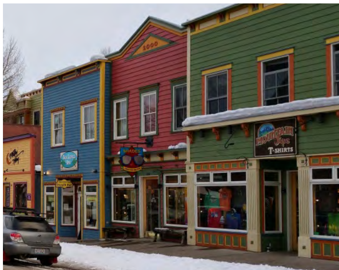
The street level of a building facing Main Street shall include a minimum of 70% transparency, have an entrance every 25-feet and be designed to provide visual interest.
