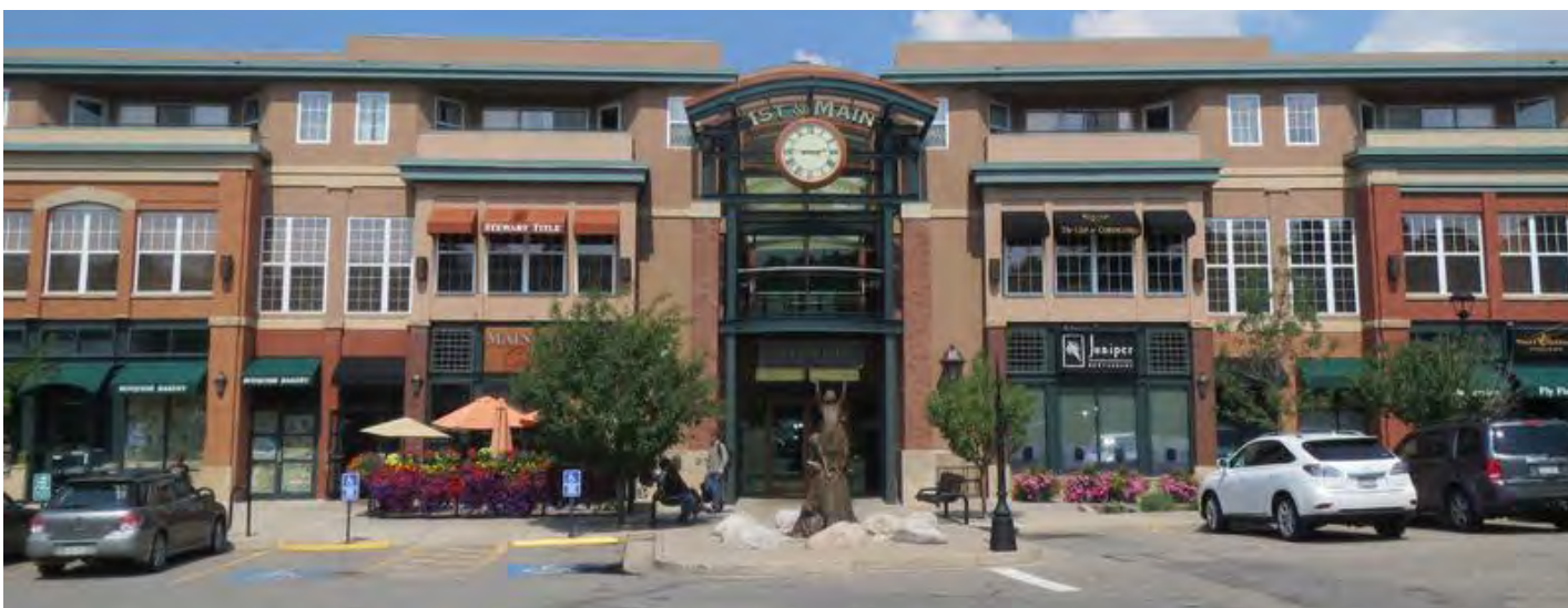
A large building reduces its mass with a traditional rhythm of storefronts, adding features like awnings and planters, and stepping back the upper level of the building. Note that this building is larger than anything that would be allowed in the 100 Block, but offers similar methods desired for breaking down the scale of a building to be human scaled.
