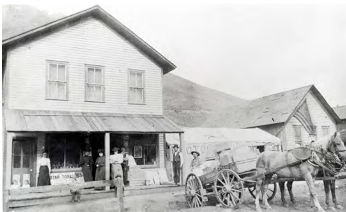
A two-story building with wood siding, sidewalks, and covered arcade includes a storefront and area where people can gather as they watch a carriage being pulled from a ditch on Main Street.
