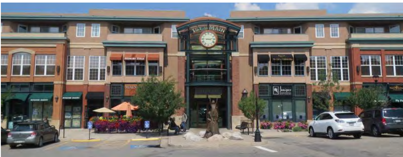
A large building reduces its mass with a traditional rhythm of storefronts, adding features like awnings and planters, and stepping back the upper level of the building. Note that this building is larger than anything that would be allowed in the 100 Block, but offers similar methods desired for breaking down the scale of a building to be human scaled.
