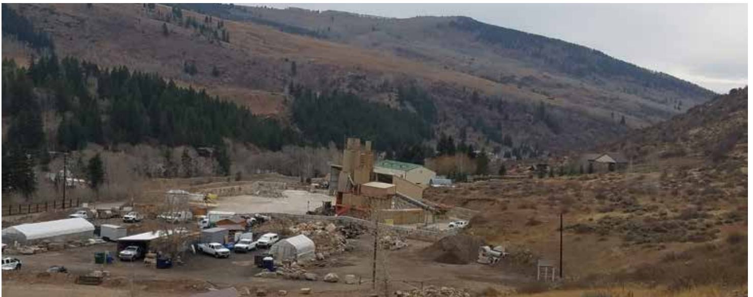
Storage Yards on Town of Minturn leased lots and the concrete batch plant and Public Works in the background.
