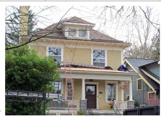
[16] The deteriorated asphalt shingles of this porch roof are being replaced in kind with matching shingles.
