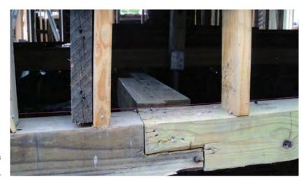
[33] Retaining as much as possible of the historic wood sill plate and replacing only the termite-damaged wood is always the preferred and recommended treatment.
