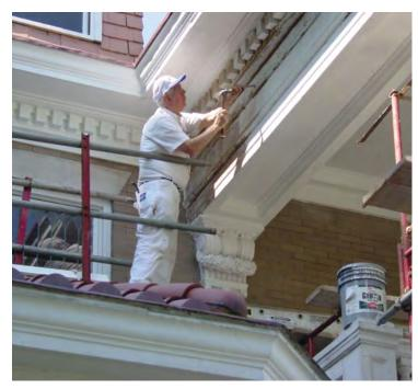
[12] Repair and limited replacement in kind to match deteriorated wood porch features is always a recommended preservation treatment.
